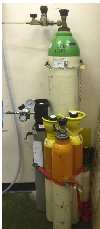
Figure 6.13 Sulphur Hexafluoride arrangement
