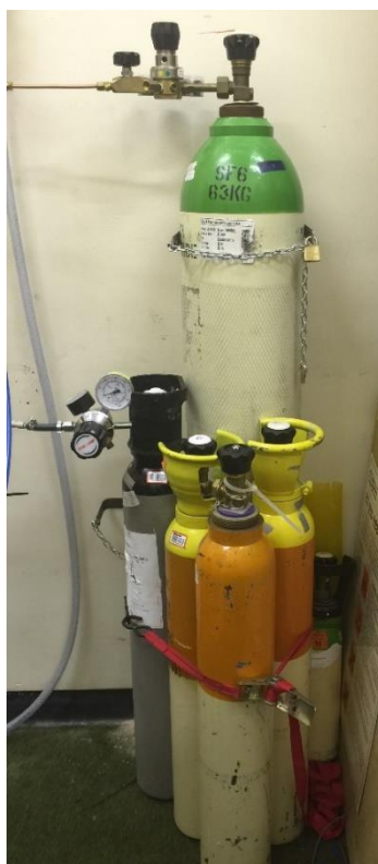
Figure 6.13 Sulphur Hexafluoride arrangement
