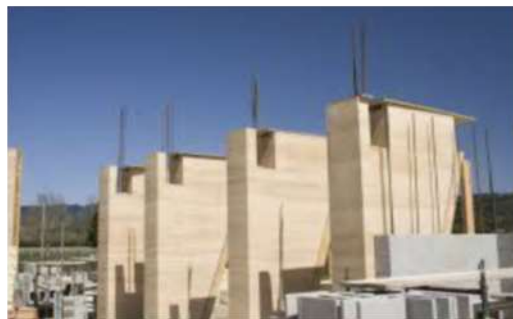
Prefabricated rammed earth panels
