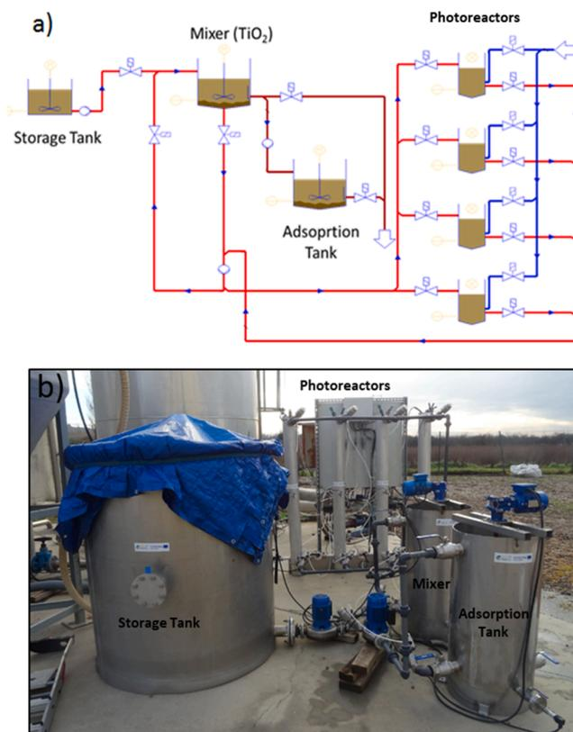
Fig. 1. 80 L/h TiO<sub>2</sub>/UV-vis and PAC adsorption pilot-scale plant: (a) process Flow diagram (b) pilot scale facility.
