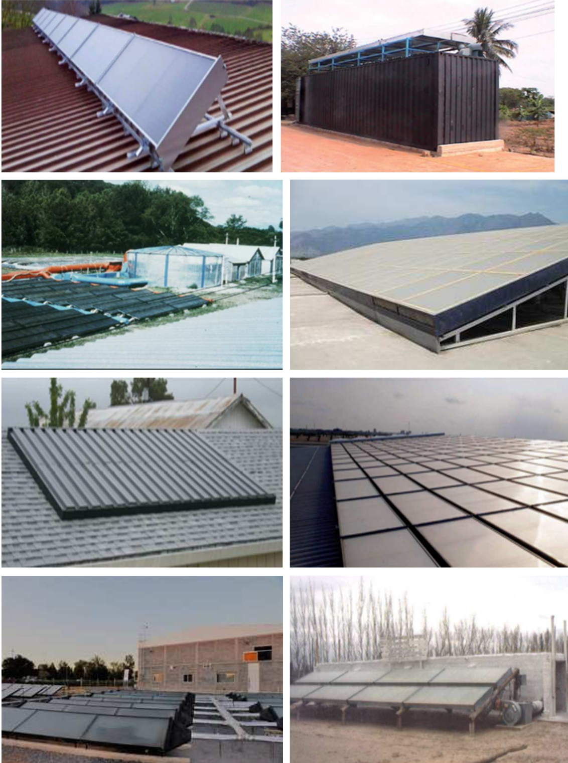
Fig.29: Various application of PV/T air collector systems in industrial processes (Ship Plants, n.d.).
