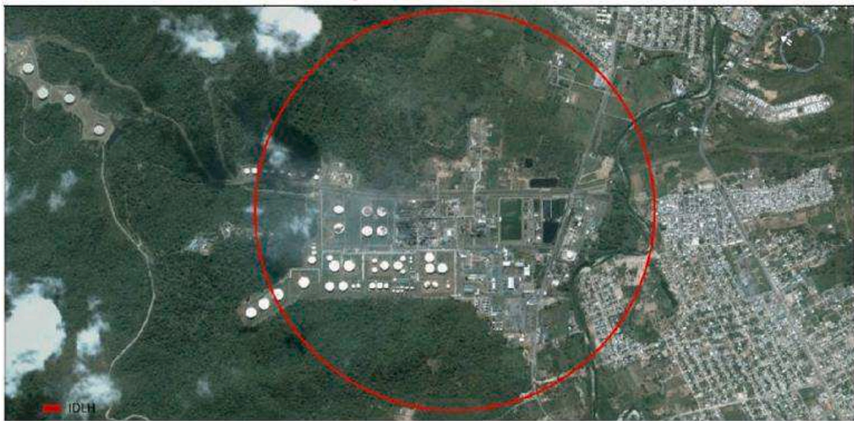
Image 6. Perimeter of immediate danger for life and health in the event of sulphur emissions from the Esmeraldas Refinery. The 50 Casas district, located in the meander of the river, is inside the circle, to the right. Source: PSRG, 2014, p56.
