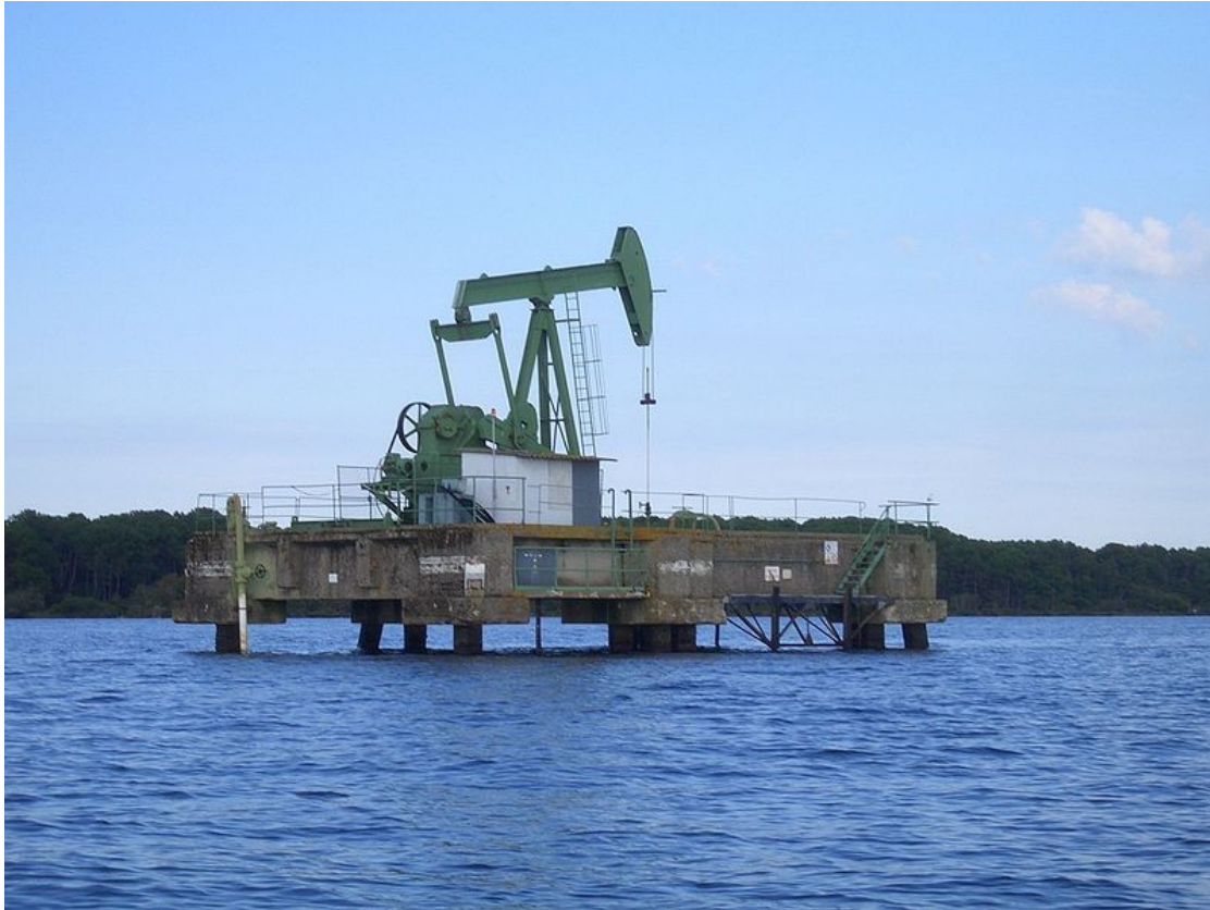
Parentis oil pumping station. © Plbcr / Wikimedia Commons, GFDL
