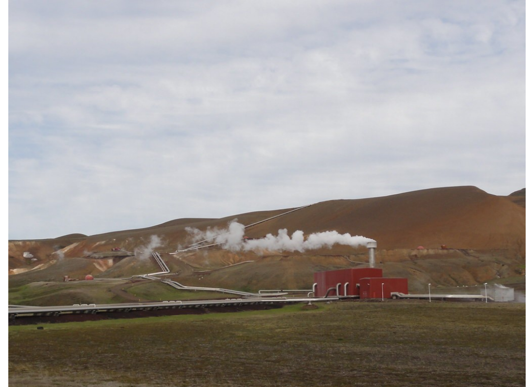
"Krafla Geothermal Power Plant" by ThinkGeoEnergy is licensed under CC BY 2.0.
